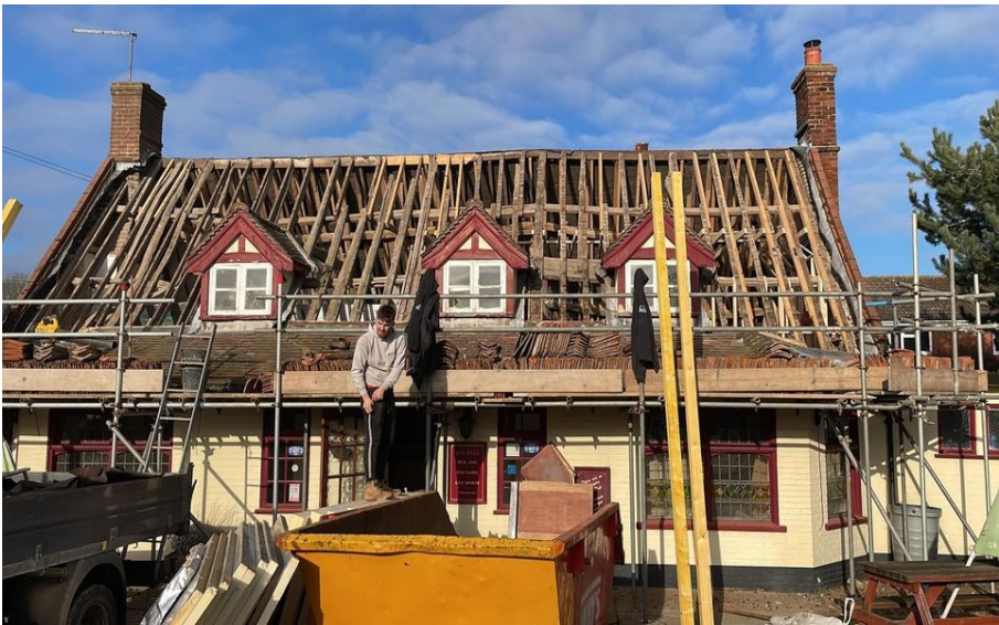
Salhouse Bell: roof replacement in progress, January 2023
